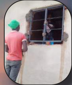
Working on the Kenyan school
